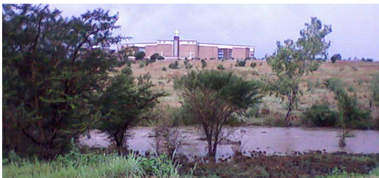
Figure 2: Kimiad stream overflowing in Moreleta Park on the afternoon of 4 April 2010
